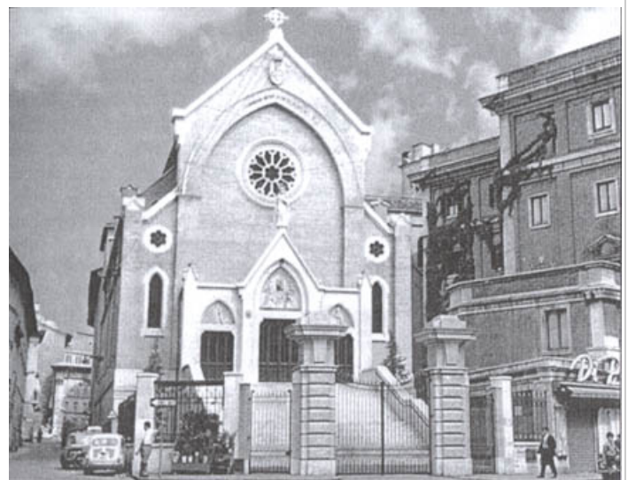
The exterior of the Church of St. Alphonsus with the international headquarters of the Redemptorist Fathers in Rome
